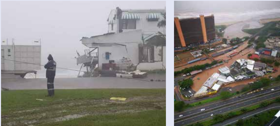
Figure 2: On the left, a collapsed house due to a mudslide along the coast, and on the right, an aerial view of flooded Amanzimtoti on 23 April 2019 (News24).
